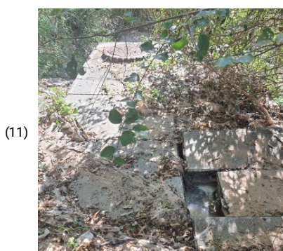
The pipe remains partially open appear partially blocked.
