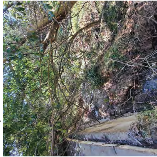
Fig. 2b. Some areas of the pipeline have been undercut and will need to be repaired.
