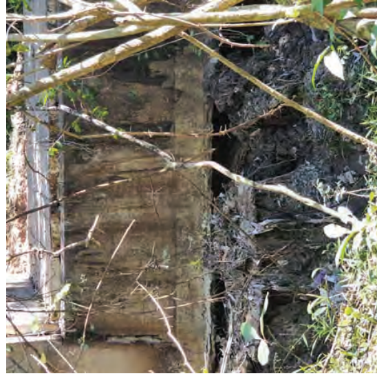
Fig. 2b. Some areas of the pipeline have been undercut and will need to be repaired.
